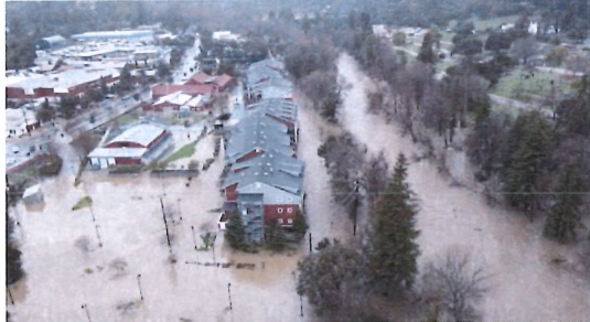
Flooding at the Tannery Arts Center
