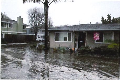
Rio Del Mar flooding on Jan. 5. (Kevin Painchaud / Lookout Santa Cruz)
