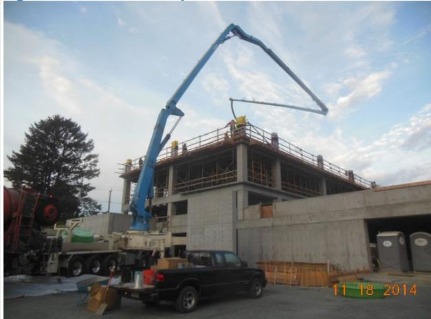
Figure 4 Concrete for Second Level
