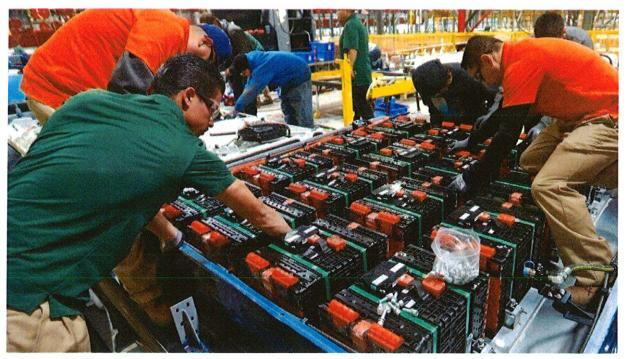
Workers install batteries on top of a bus destined for UC Irvine. BYD's business began with production of cellphone batteries. (Mel Melcon / Los Angeles Times)
